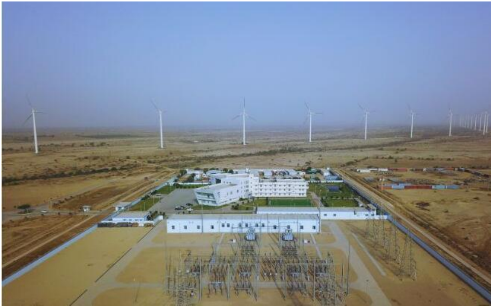
Aerial View of the Second Wind Farm
