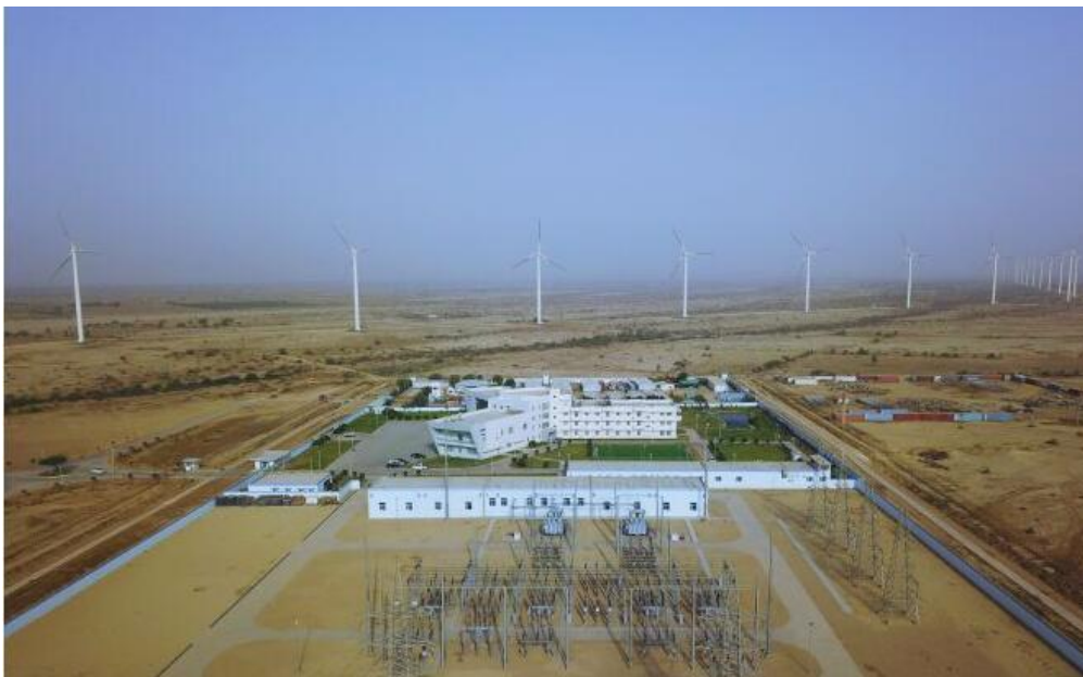
Aerial View of the Second Wind Farm
