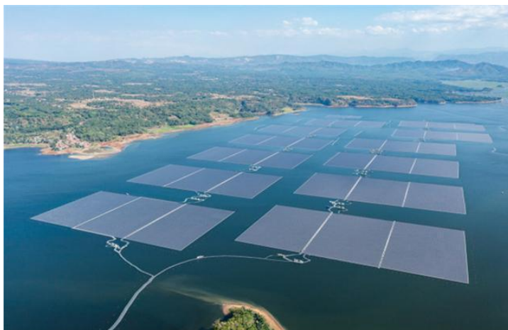
Figure 7 Overall View of the Cirata Floating Solar Photovoltaic Power Project
