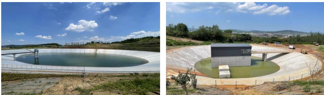
Figure 3 On-site view of the distributed pumped storage power station in an abandoned mine shaft
