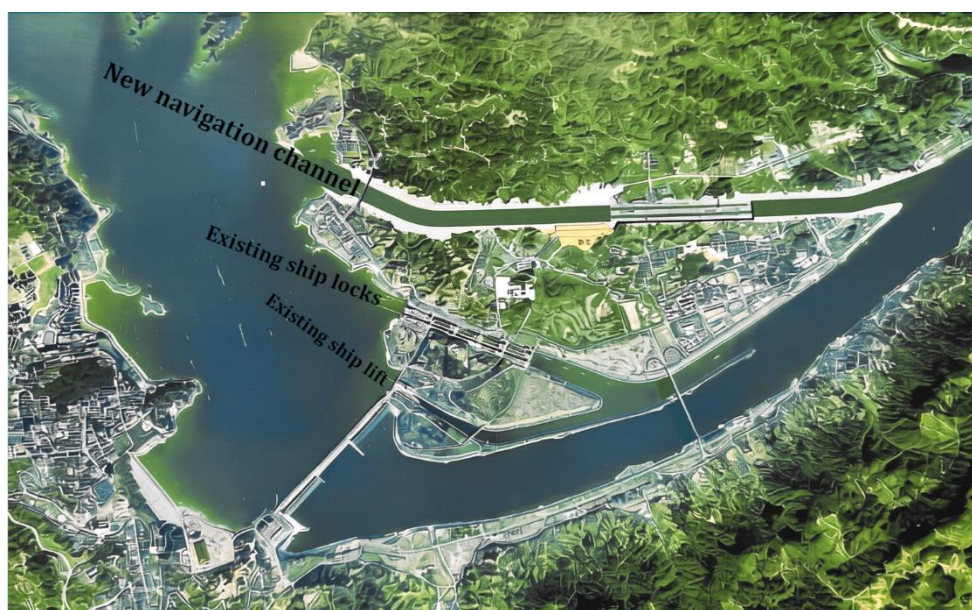
Figure 3-7. Existing Three Gorges ship locks and the new navigation channel (under construction)
